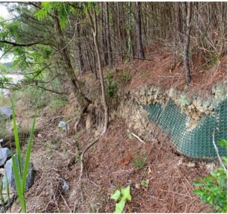
Figure 4. Example of fastland erosion at base of embankment.
