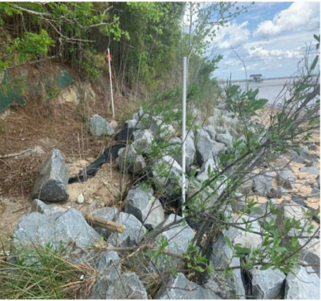
Figure 2. Riprap from failed revetment on the beach.
